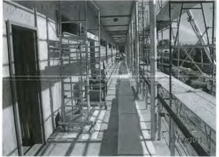
2 ND FLOOR EXTERIOR DECK
