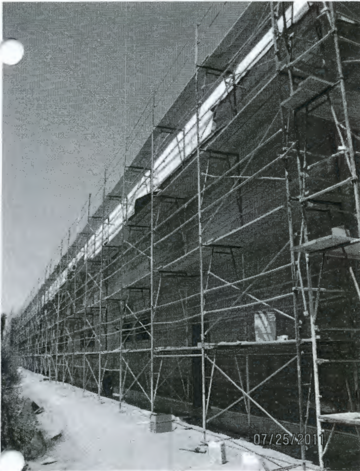
EXTERIOR BUILDING ENCLOSURE
